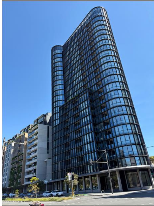
Figure 1: 28 Zetland Avenue, 77-93 Portman Street and 32 Ebsworth Street, Zetland, viewed from the south-east
